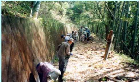
Maintenance of canal
